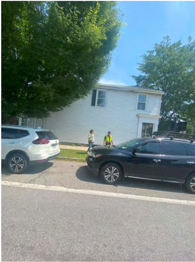
Photo 45 - #1 Chatham St. (from Albany Ave.), Built 1850
