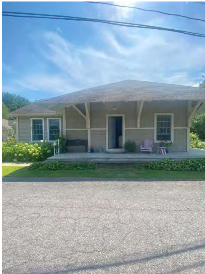
Photo 28 - #36A Railroad Ave. (from Railroad Ave.), Built 1998
