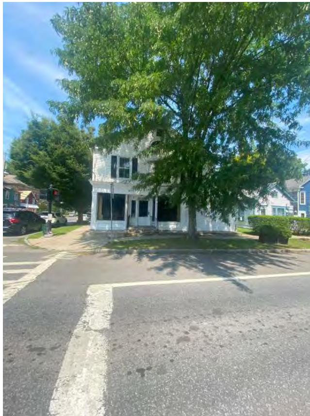
Photo 46 - #1 Chatham St. (from Chatham St.), Built 1850
